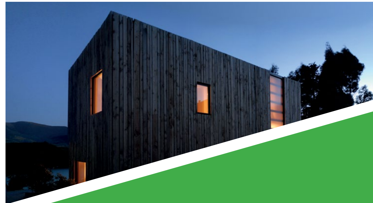
The Warrander Studio, a house project designed and built as part of the SARC 591 Master of Architecture (Professional) Thesis, by Ben Sutherland.
